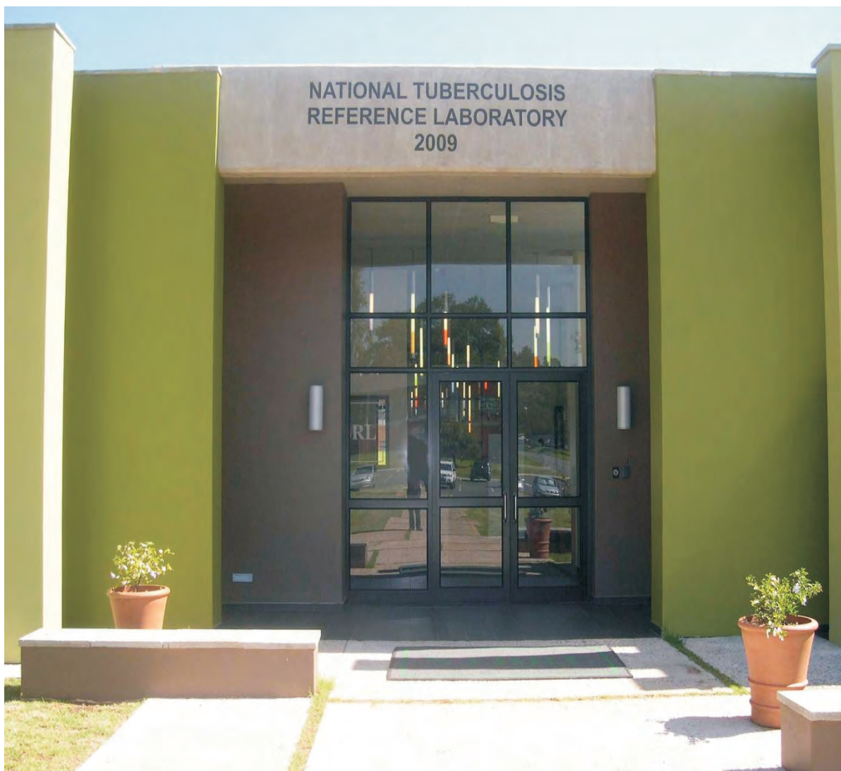
Entrance to the new National TB Reference Laboratory at Sandringham, Johannesburg
